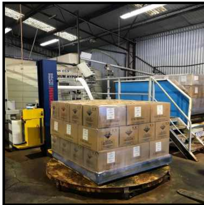
SODIUM HYPOCHLORITE PLANT AUTOMATIC STRETCH WRAPPING MACHINE
